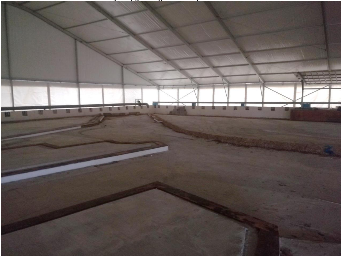
Picture 4: Wave bassin after major upgrade (post-2018)
