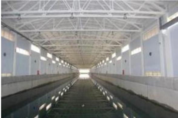
Figure 3 Multifunctional Ship Model Towing Tank
