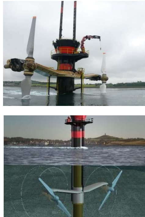
Figure 7. The Seagen 1.2 MW device operating at Strangford Lough, Northern Ireland (U.K.).
