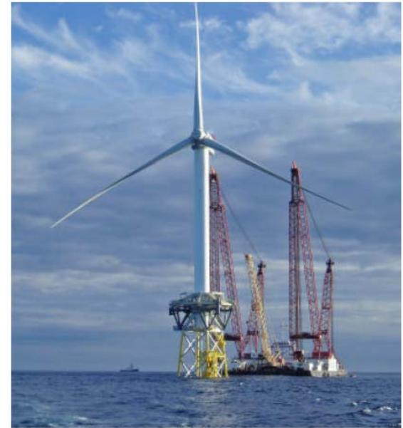
Fig.1: Installation of a 5 MW Turbine on Jacket Substructure (Source: REpower Systems AG)
