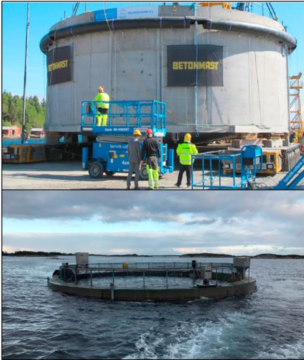
Figure 190: Concrete containment fish tank (Picture courtesy of Tor Ole Olsen).
