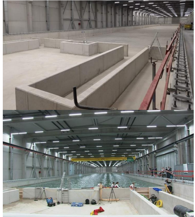
Figure 84. Top: view from the dock section of the new towing tank at FML (Delefortrie et al., 2019). Bottom: status January 2021. Due to COVID-19, the basin is being used as a training centre for the Belgian Olympic kayak team. (©Sporza.be).
