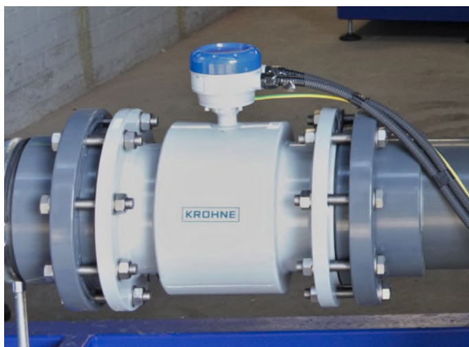
Figure 4: Magnetic flowmeter situated at the lower limb of FTFC.
